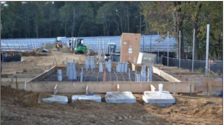
***Above:** This will be a concrete pad for the DC to AC inverter and SMECO's transformer. There will be six of these pads in the solar plant. **Below:** Solar panels that have been installed.*
