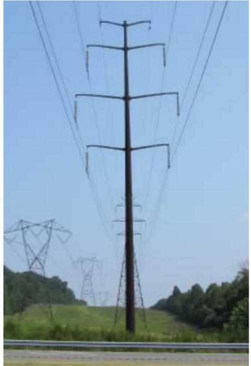
*This is an example of a similar double-circuit 230-kV pole located in Reston, VA. This pole is approximately 110 to 130 feet and is the same self-weathering (brown) steel as SMECO's poles.*
