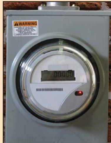
← *Advanced meters will be solid state similar to the meter pictured at left. AMI will capture detailed kilowatt-hour usage information, enabling customers to manage energy usage.*
